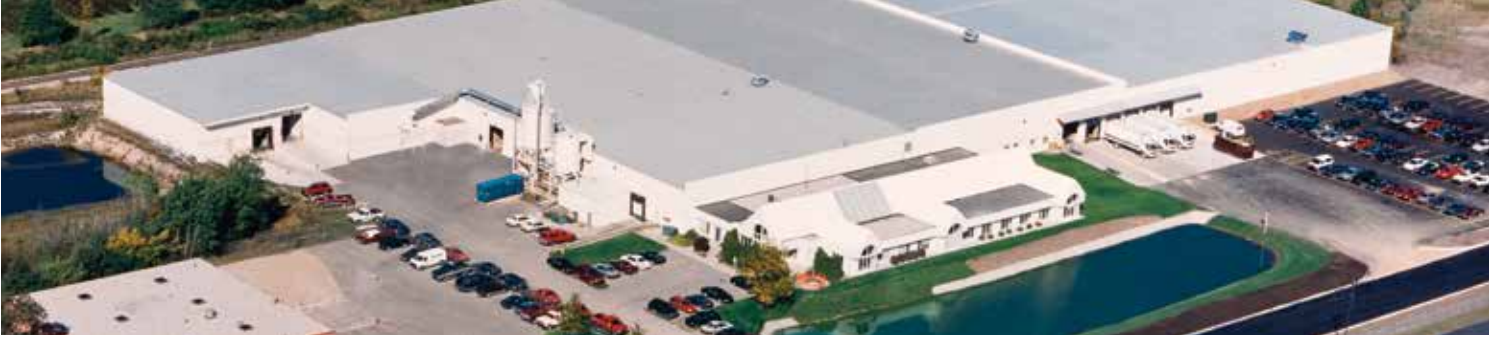
Our 200,000-sq. ft. manufacturing facility in Holland, Michigan.
